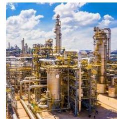
Oil & Gas Plant
